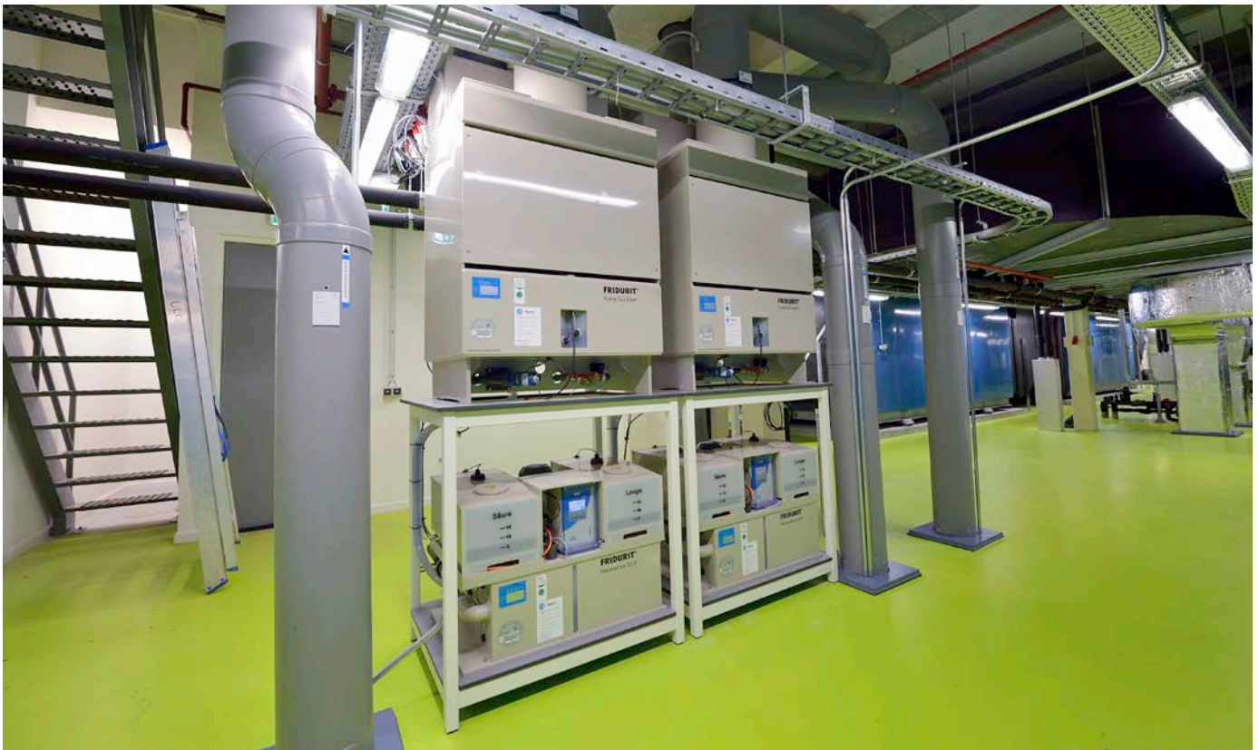
FRIDURIT fume scrubber C180 with FRIDURIT neutralisation unit for the treatment of the contaminated waste-water from the fume scrubber.
